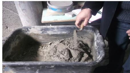
**Figure 1.6:** concrete after fully handmade mixing
